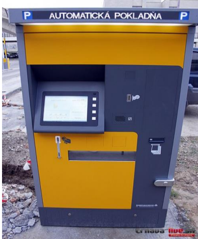
Figure 9 Automatic parking ticket office for P+R Poprad – Tatry
